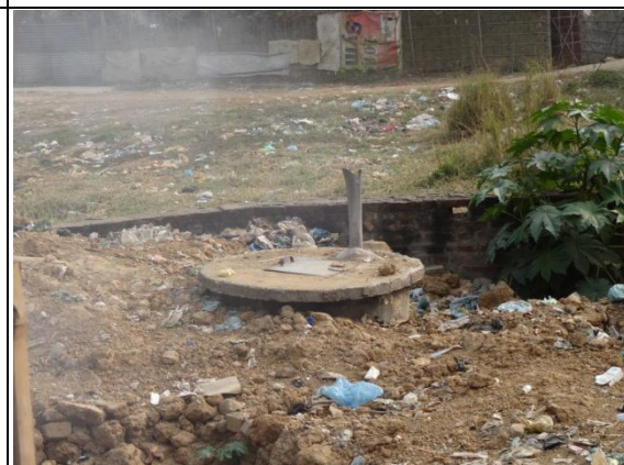
Pit for sharps at Dimapur Dist. Hospital
