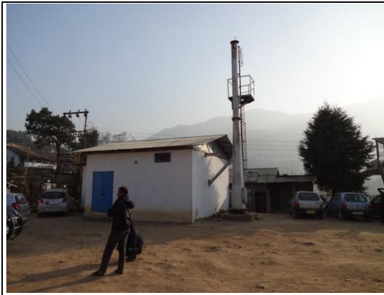
Non-functional Incinerator at Naga Hospital at Kohima
