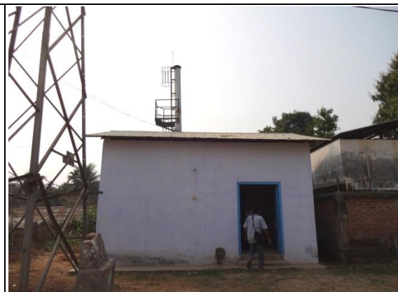
Incinerator at Dimapur District Hospital
